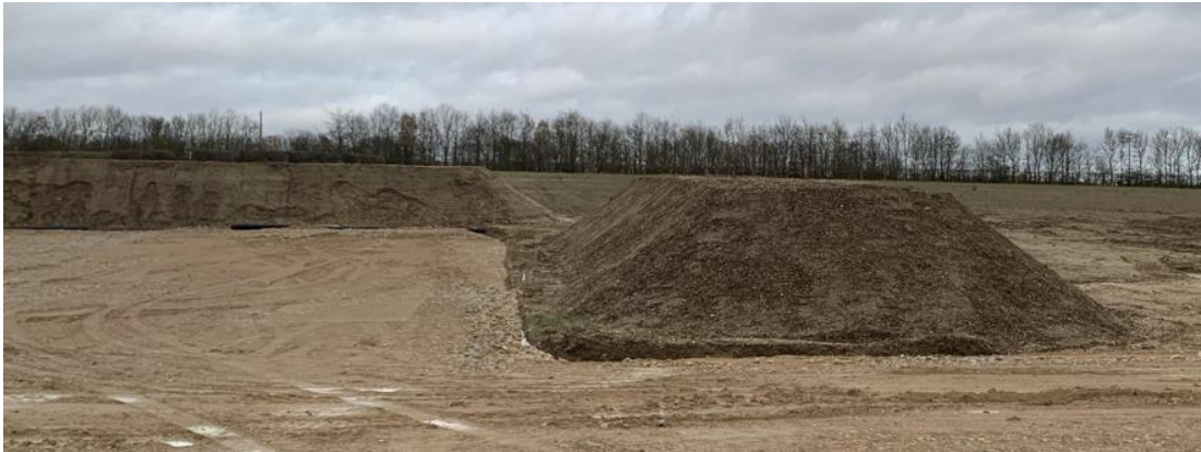
Photo 14: Topsoil Storage Example
