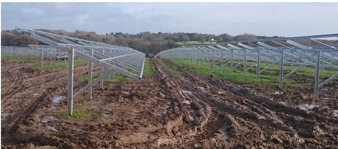
Photo 4: Soils not Suitable for Trafficking
