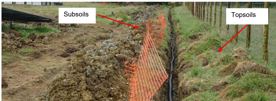
Photo 26: Subsoils Dug out of the Trench
