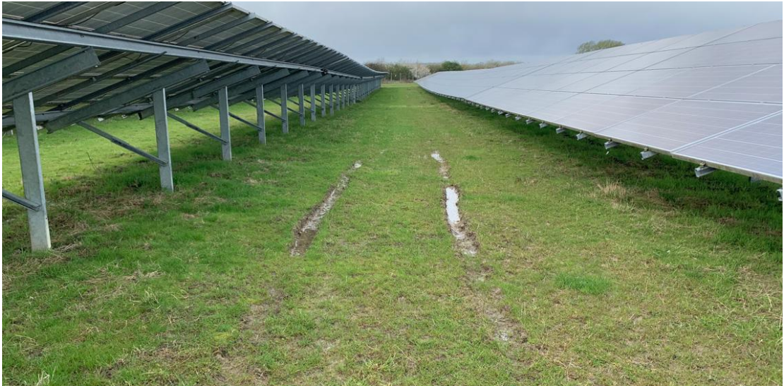
Photo 33: Ruts Caused by Vehicles
